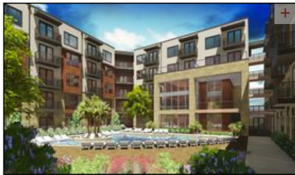
Artists rendering of the Lenox Boardwalk project that has broken ground at South Pleasant Valley Road and Elmont Drive in Austin. Credit: ... Read More
